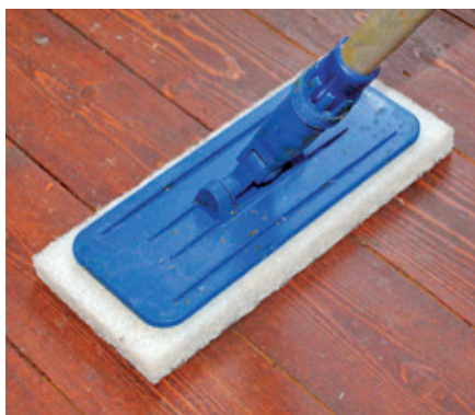
Linseed Oil Wax applied easily with rough scouring pad type Scotch Brite.
