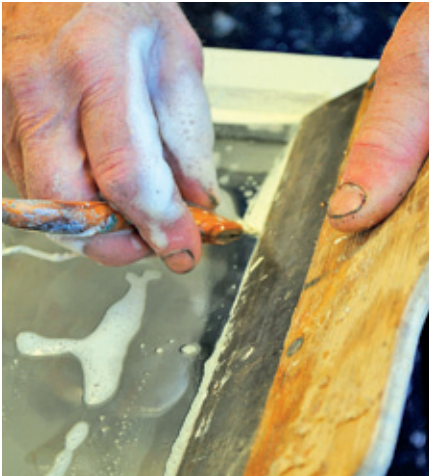
Cut the edges of the putty rebates in slightly soapy water.
